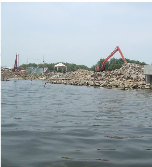
Fig 13. Construction of the seawalls
