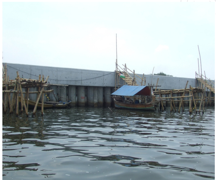
Fig 14. The giant seawalls
